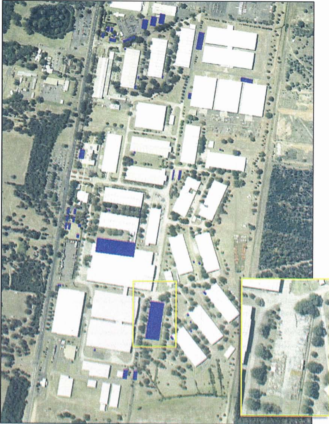
Figure 20: Locations of former buildings (purple) in undeveloped areas of the DNSDC (based on a 1966 plan of the site). Inset shows surviving slab of former store building. Base map – Google Earth.
