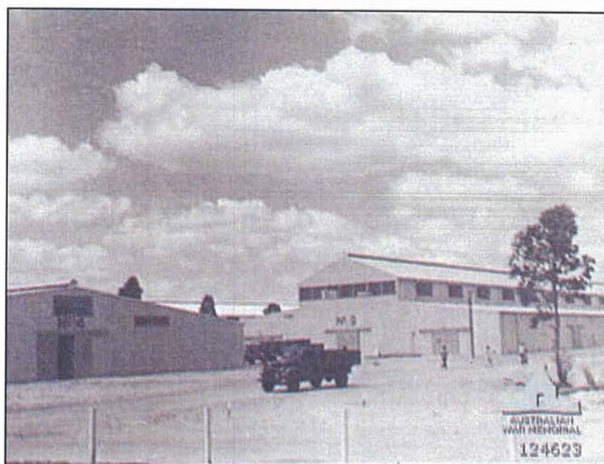
Figure 10: 5th Aust. BOD exterior view of No. 9 Bulk (Crane Served) Technical Store Shed, 23/1/46 (Source: AWM, ID No. 124623)
