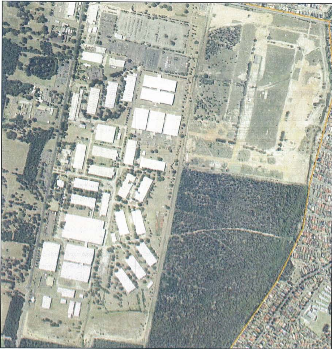
Figure 12: Current aerial photograph of the DNSDC (Six Viewer).
