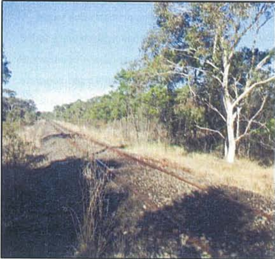
Figure 44: Existing rail link running through vegetated area. Facing south-west.
