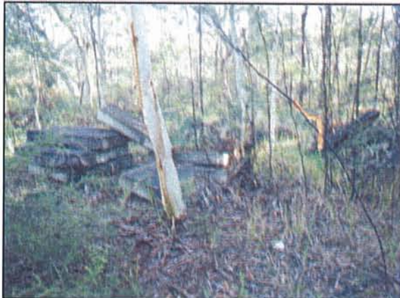
Figure 46: Slabs of concrete and other structural material within vegetated area.
