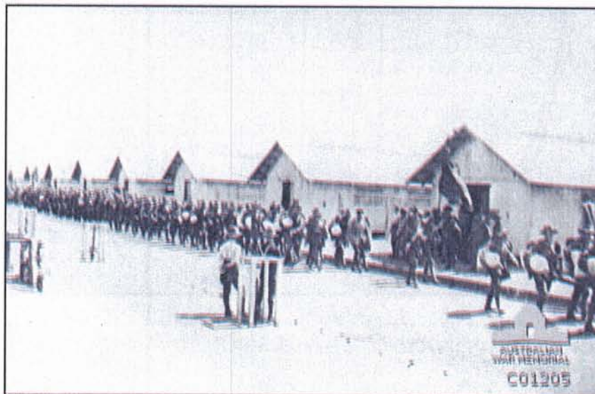
Figure 3: Accommodation huts, Oct 1916 (Source: AWM, ID No: C01205)
